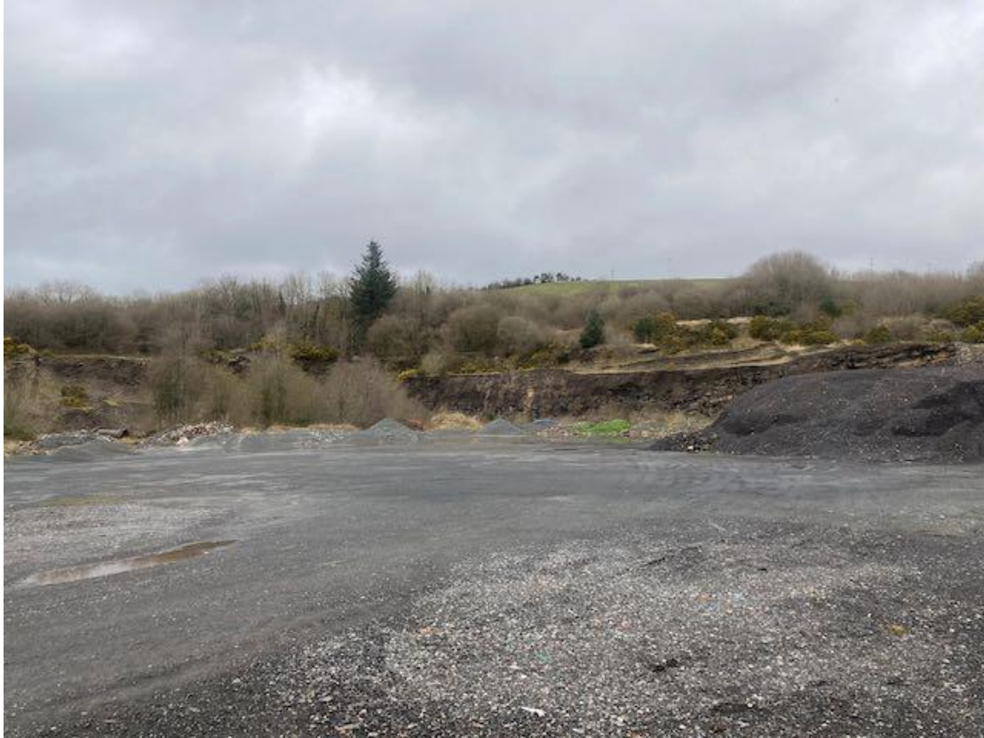
Main works area at Glenmore Quarry
