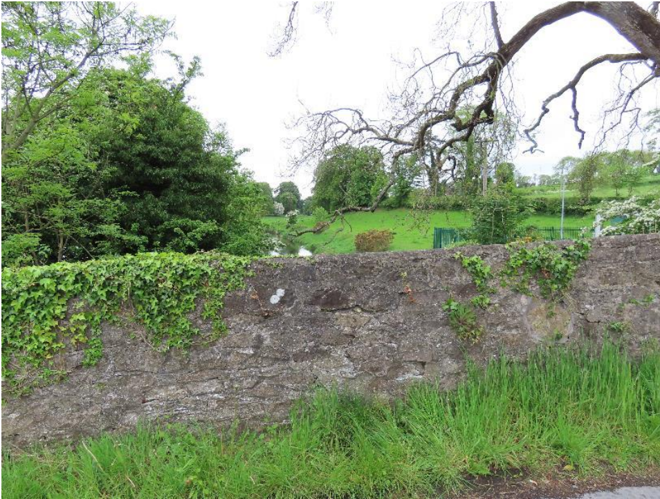
Plate 4-3 - Upstream Parapet Wall
