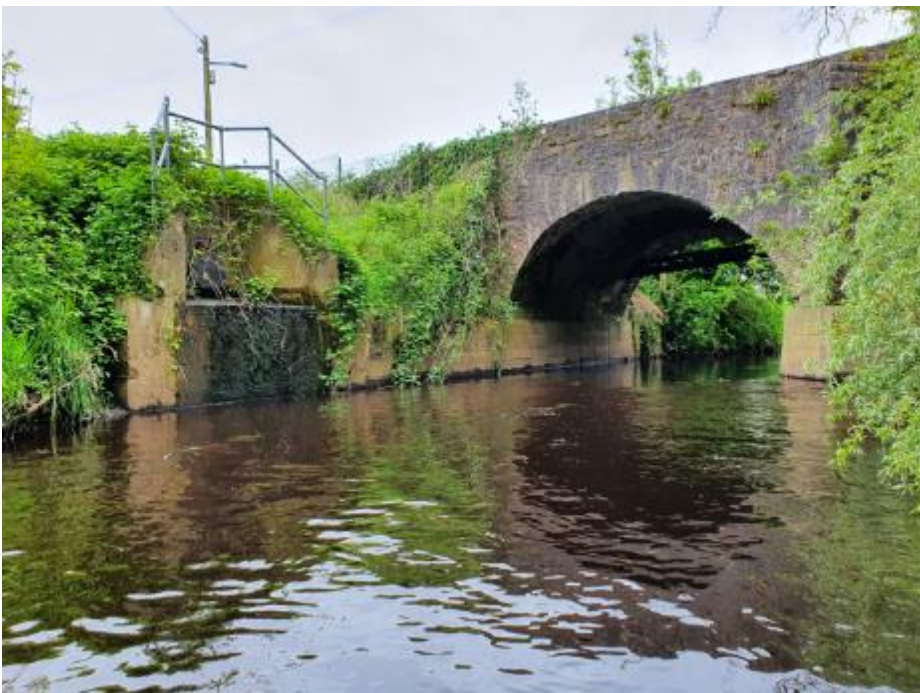
Plate 4-12 - Downstream elevation of western arch
