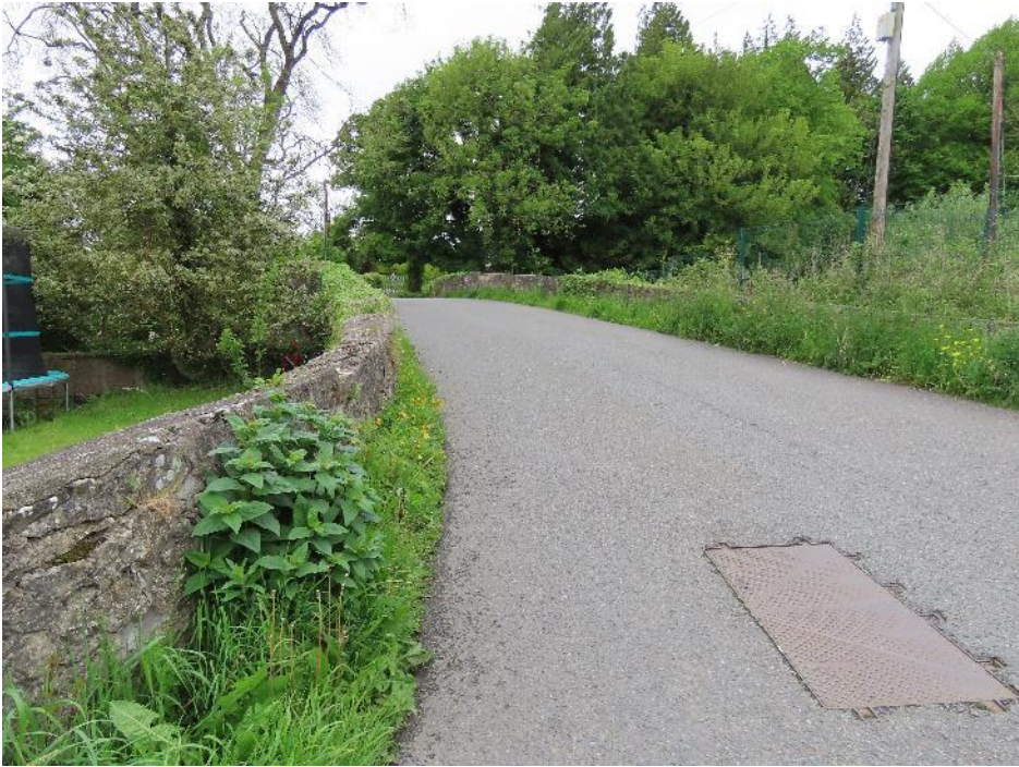
Plate 4-1 - Ballyalbany Bridge - Looking Northeast
