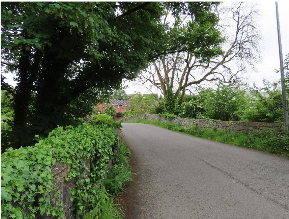
Plate 4-8 - Looking southwest over Ballyalbany Bridge. Mature ash beside bridge with ash die-back disease
