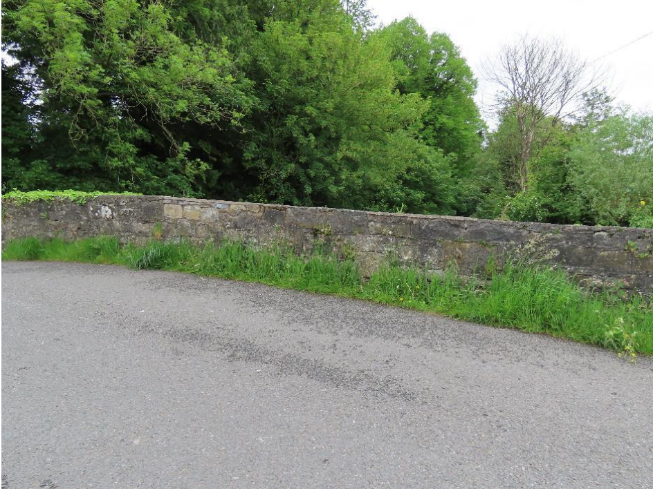
Plate 4-2 - Downstream Parapet Wall
