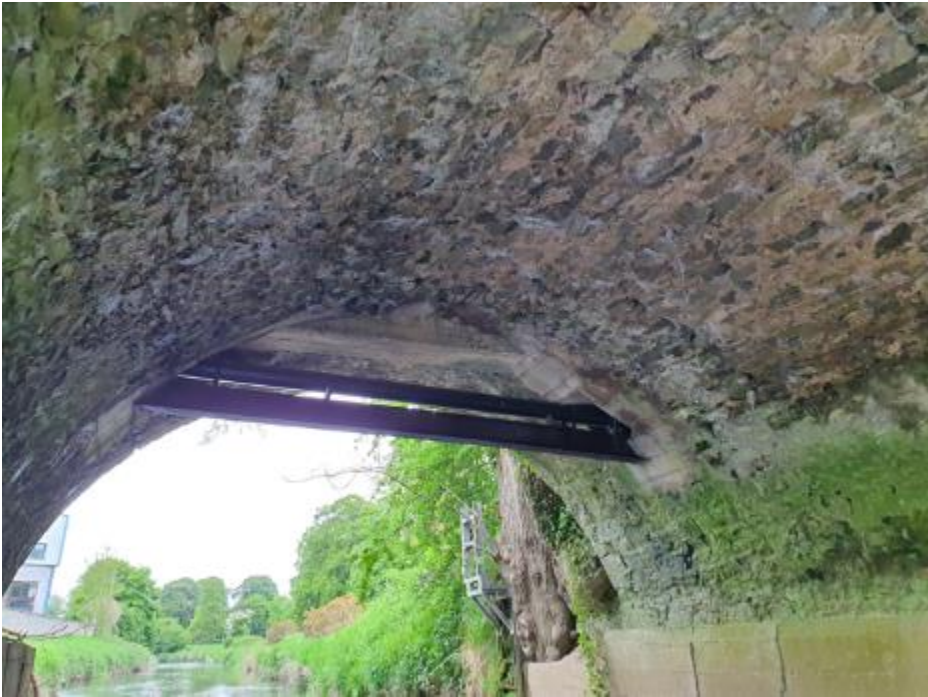
Plate 4-13 - View under eastern arch - no crevices suitable for retention for bats
