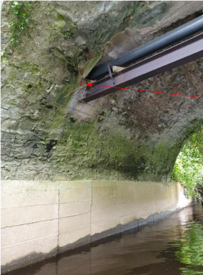
Plate 4-17 - Active Dipper's nest on metal girder under eastern arch
