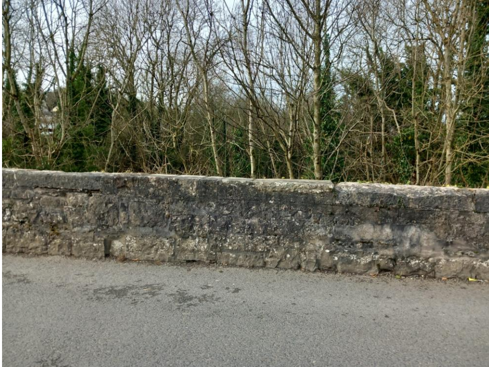
Plate 12: Detail of bridge wall
