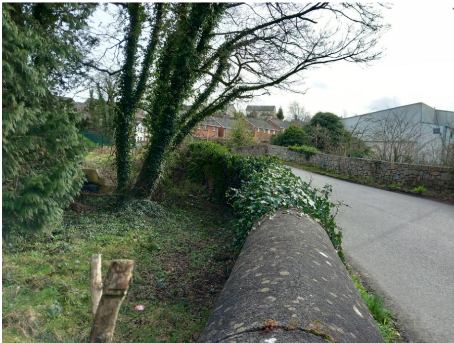
Plate 3: Rounded capping detail
