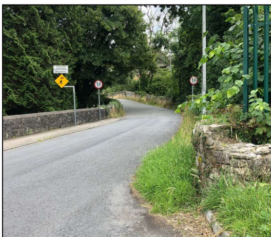
Figure 1-1 – Existing Ballyalbaney Bridge
