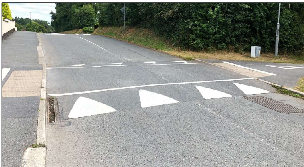
Figure 3-5 – Existing Ramp and Utility Chamber
