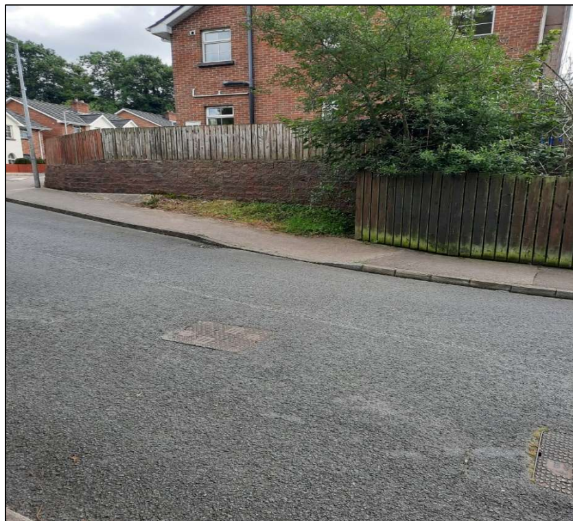
Figure 2-1 – Existing drop kerb
