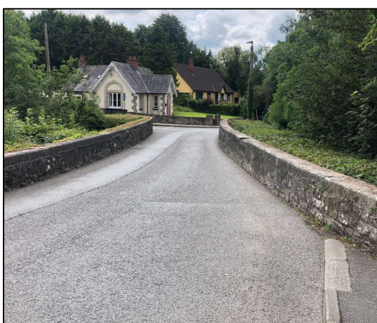
Figure 1-2 – Existing Horseshoe Bridge
