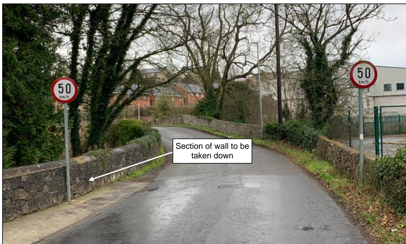
Figure 5-5 - North side of existing bridge (facing south)
