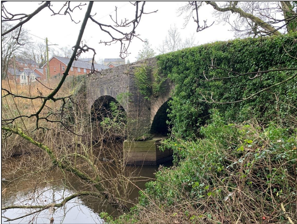
Figure 4-6 - Ballyalbany Bridge east elevation
