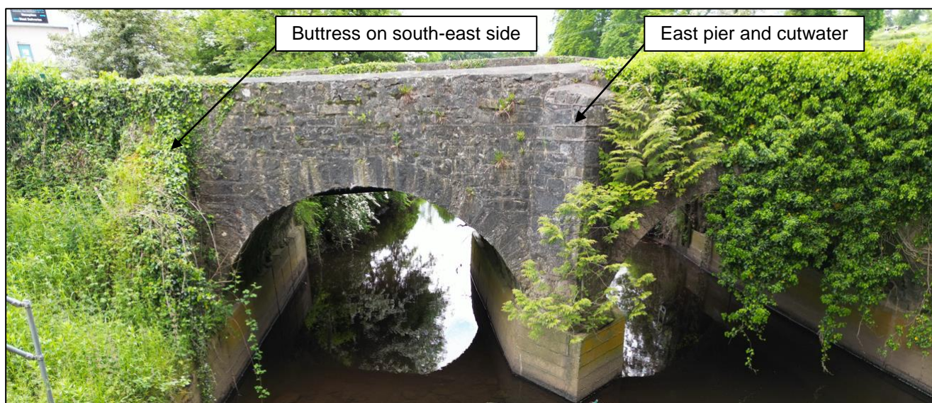
Figure 5-3 - East elevation of existing Bridge
