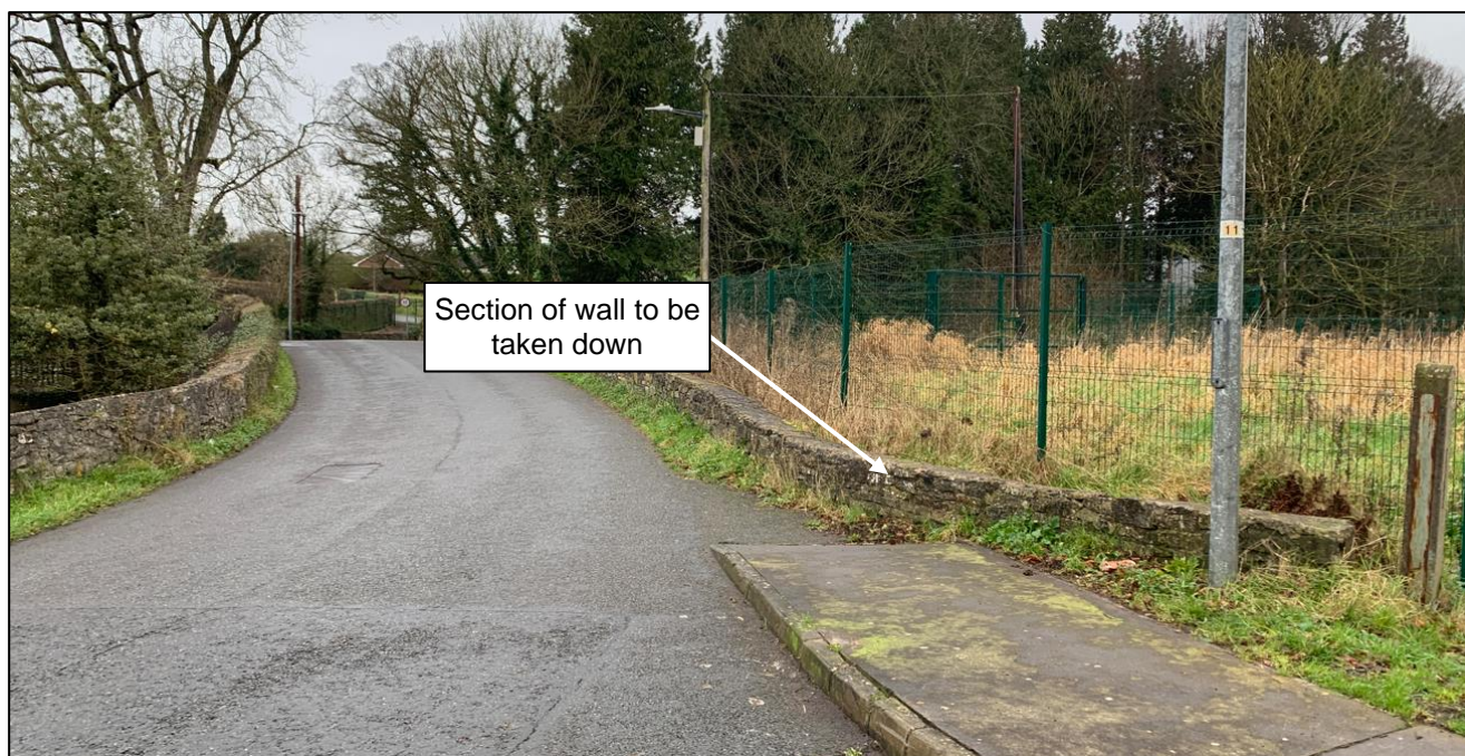
Figure 5-4 - South side of existing bridge (facing north)
