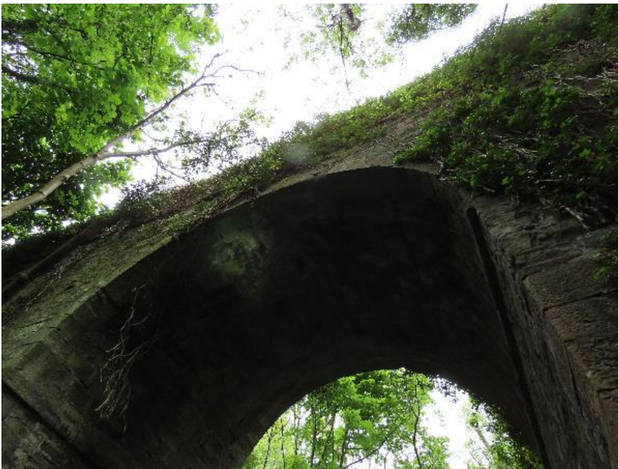
Plate 4-10 - Under surface of arch
