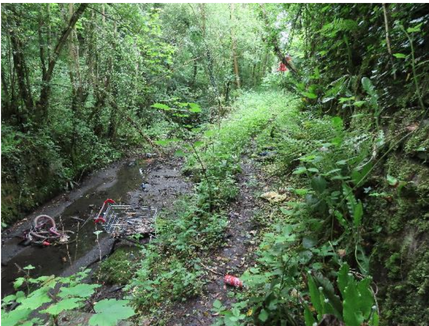
Plate 4-12 - Looking east along tow path. Rubbish in channel
