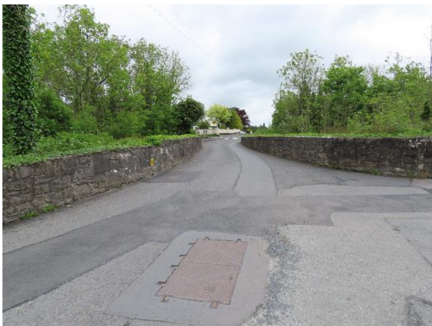
Plate 4-2 - View across bridge looking north
