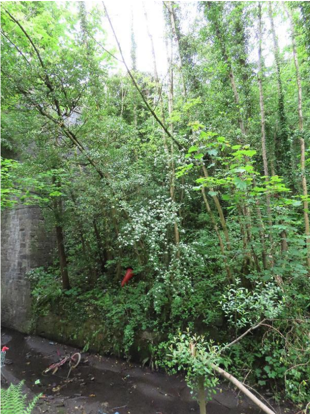
Plate 4-17 - Ash and sycamore saplings on northern embankment to east of structure
