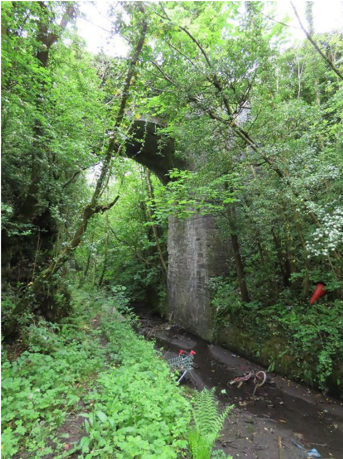
Plate 4-16 - Eastern elevation of bridge from tow path
