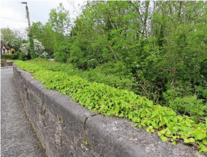
Plate 4-3 - Cut stone parapet walls with considerable ivy growth
