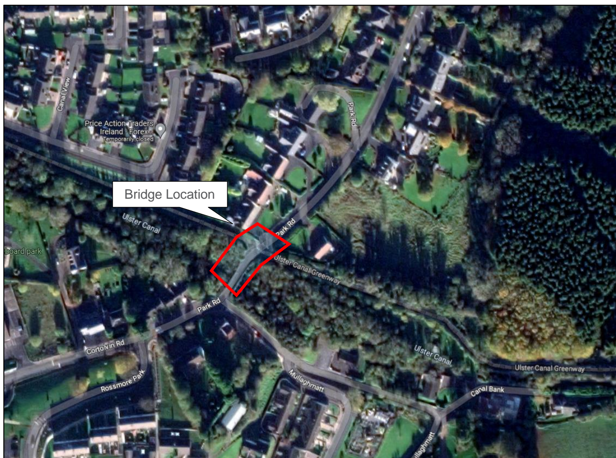
Figure 1-1 - Location of Horseshoe Bridge
