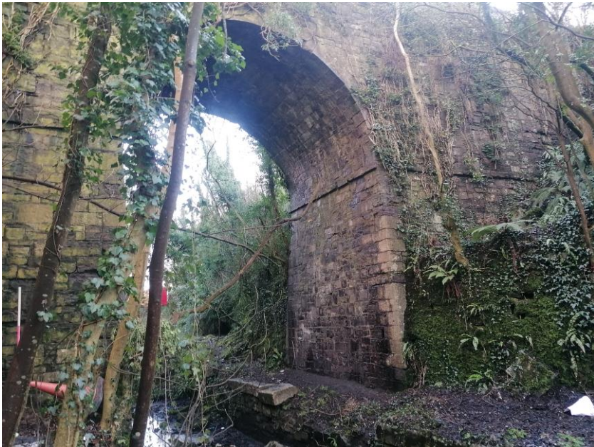
Plate 7: Horseshoe Bridge, Note tug path passing under bridge on south side
