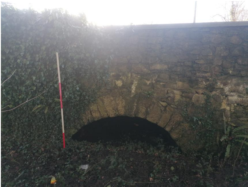
Plate 3: Ballyalbaney Bridge, smaller third arch within southern graveyard grounds near riverbank
