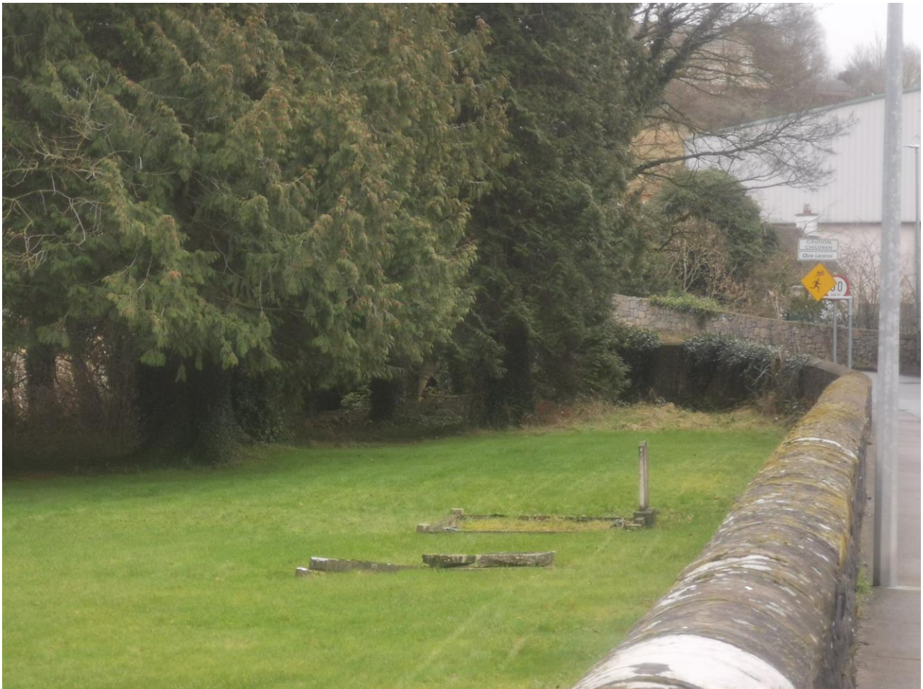
Figure 1: Picture of the survey area with the Ballyalbany Bridge in the background (looking south)
