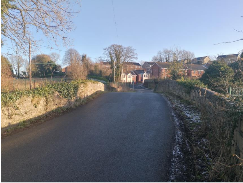
Plate 1: Ballyalbaney Bridge, facing SE, wide enough to allow 2 cars, note the hump
