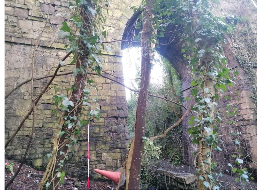
Plate 6: Western face of Horseshoe Bridge, Note height of arch
