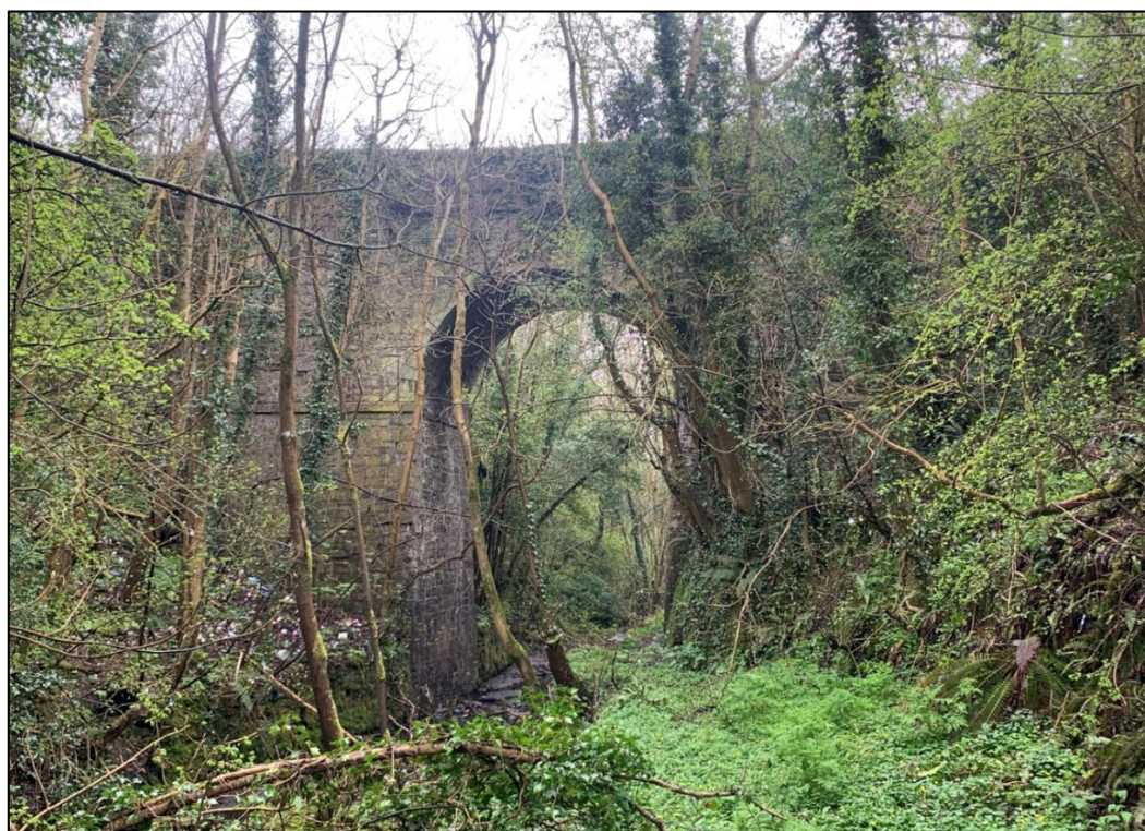
Figure 4-6 - Horseshoe Bridge west elevation
