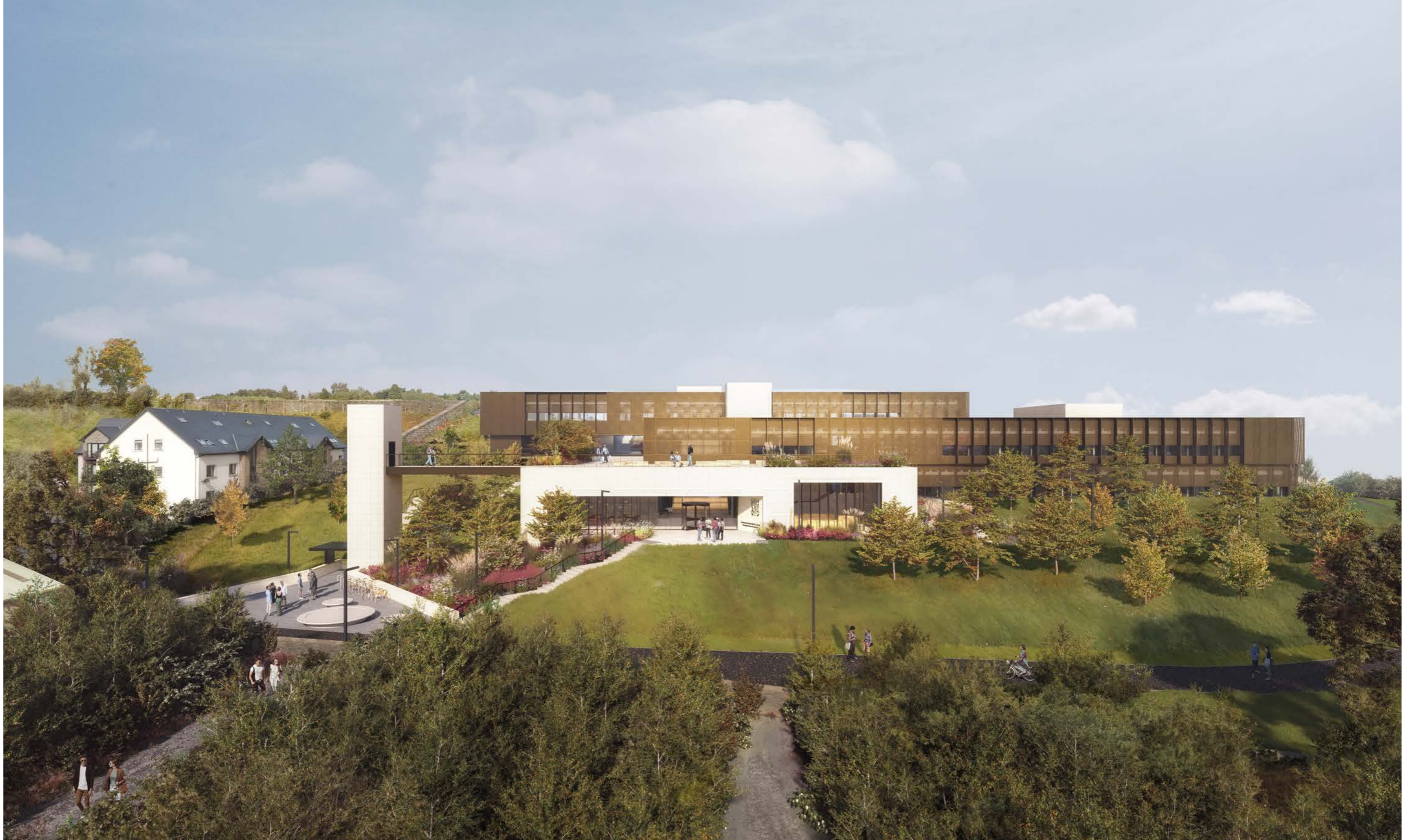
Aerial View from Dublin Street North
