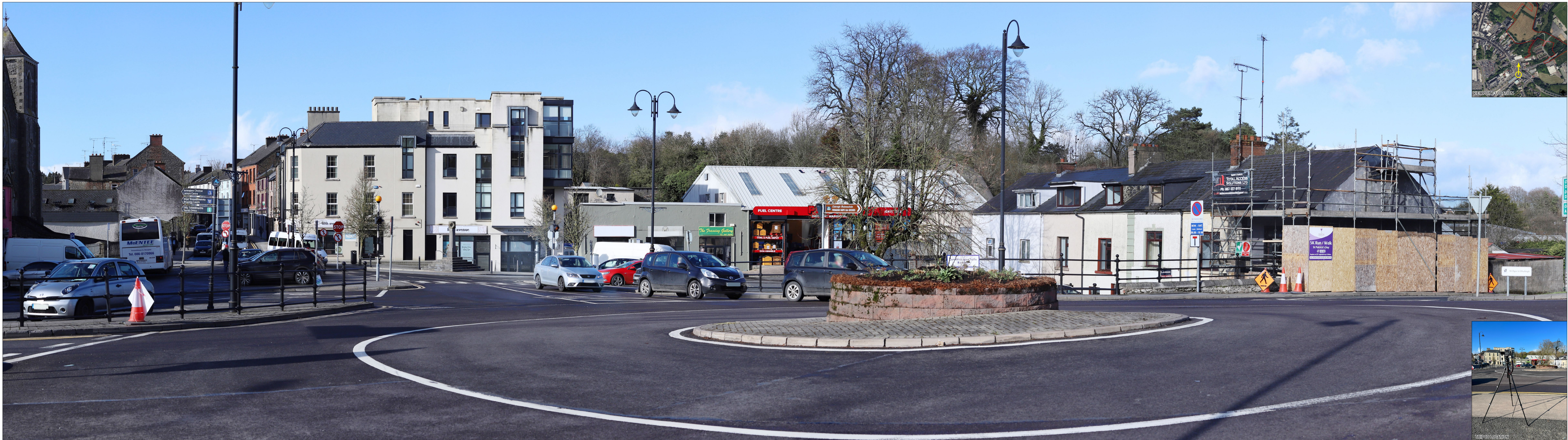
EXISTING BASELINE VIEW
