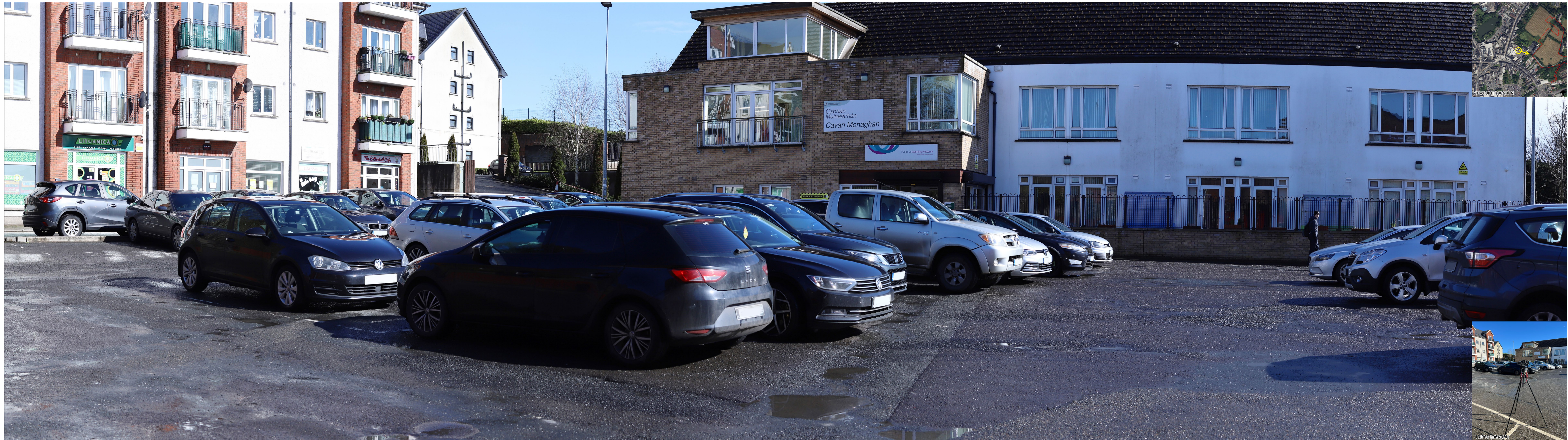
EXISTING BASELINE VIEW
