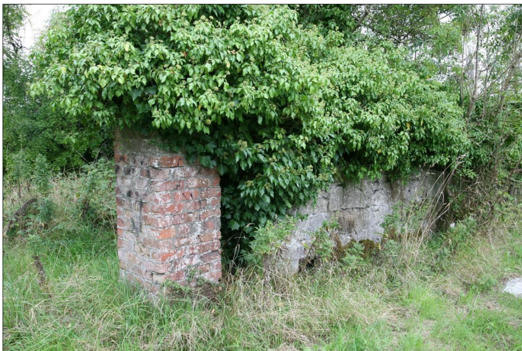
Plate 2 Brick pier terminating eastern precinct wall, Area 1
