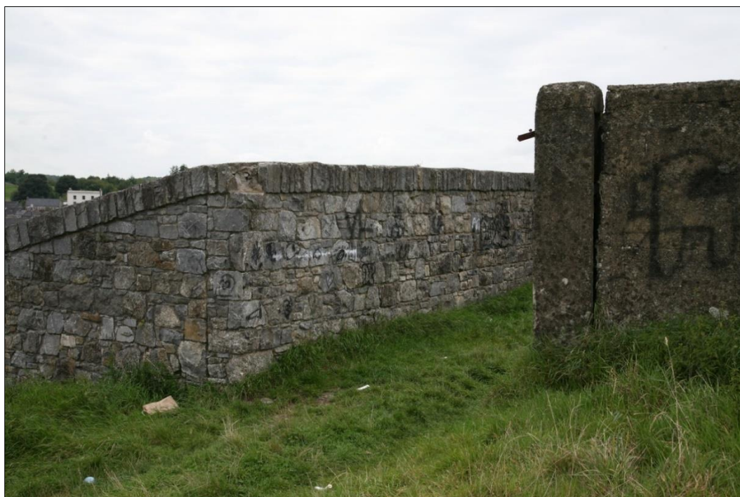
Plate 6 Entrance from Area 2 to Area 4. Note different types of walling
