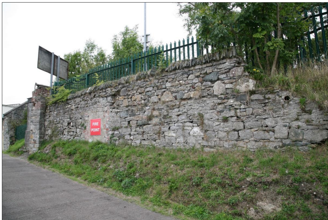
Plate 3 Exterior view of southern precinct wall, Area 1
